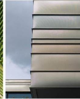
Horizontal Zinc Cladding
